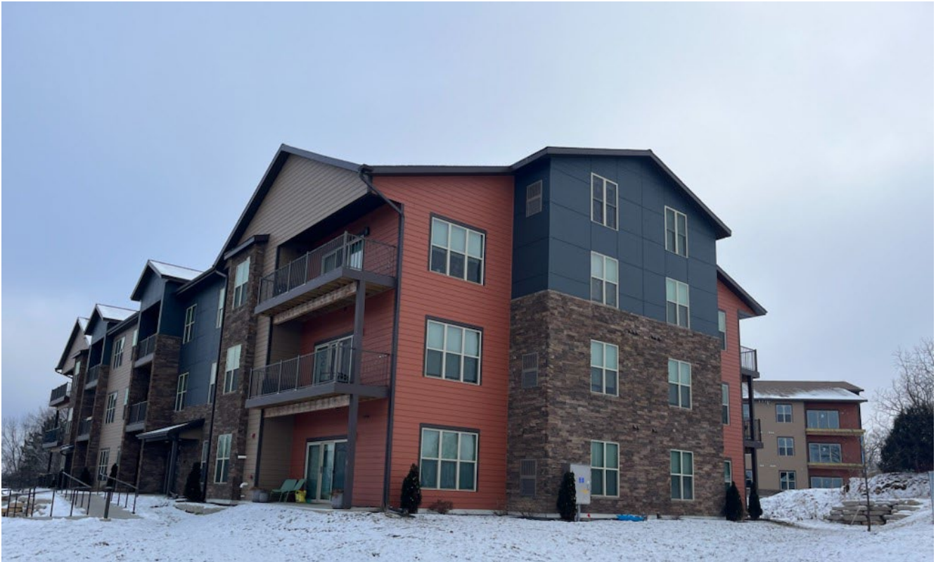
Figure 2: Waubesa Village - end view
